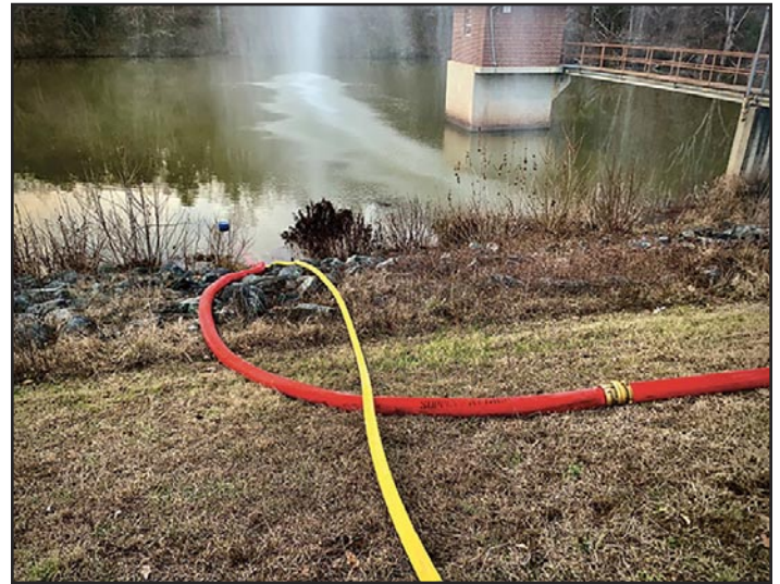
5 To work effectively, no more than 100 feet of 5-inch hose should be used with the TurboDraft. This will yield the desired water flow return ratio to make this device effective in the rural environment.
