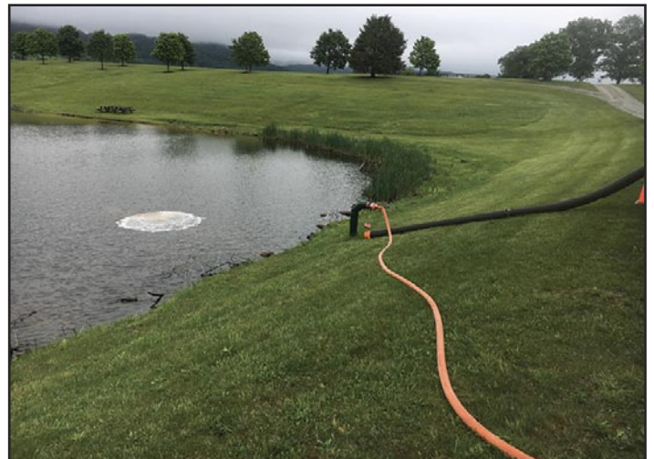
3 When using a dry hydrant to access distant water sources, it is critically important for the operator to flush the hydrant prior to attempting to draft.
