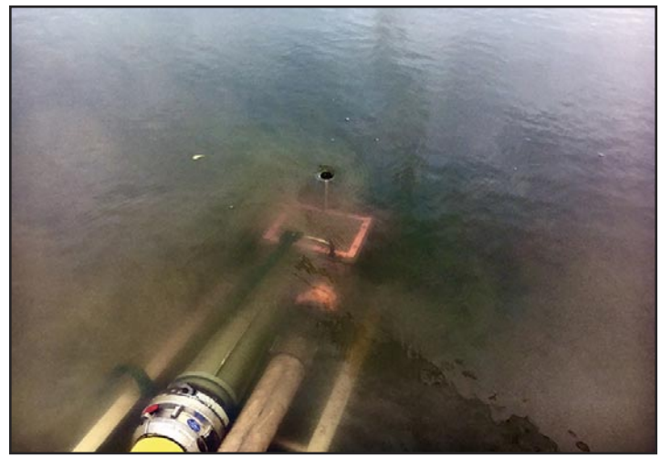
6 The TurboDraft pictured here was secured to a ground ladder and then pushed into the source. Since this source had a shallow bank, it caused the ladder to dig into the bank and limited how deep the TurboDraft was submerged. This caused a whirlpool to form during the operation, which limited flow.
