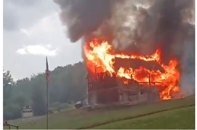
Fire crews were met with extreme fire conditions
