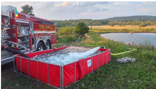
5" LDH secured to frame tank creating the "open relay" for the fill site.
