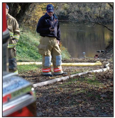
A lift of about 20 feet through 150 feet of hose was no challenge for the TurboDraft, which produced about 300 gpm of useable flow in this evolution.
