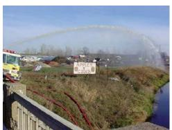
Figure 16. This department is using a single engine to supply two TurboDrafts (into a stream), which are supplying the pumper with a net flow of 932 gpm.
